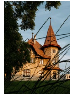
M.A.D House Exterior view
