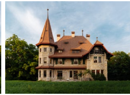
M.A.D House Exterior view
